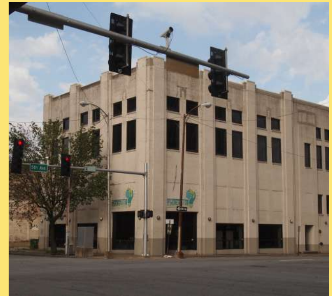
The Generator. ©CORI
