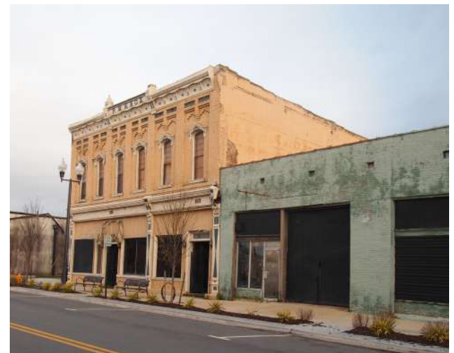
Many buildings in downtown stand empty. ©CORI
