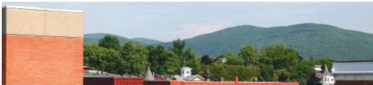
The views from the top floor of the parking garage are some of the best in downtown Rutland. ©CORI
